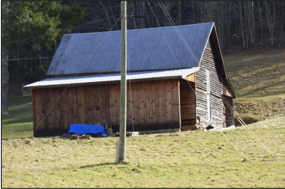
Photo 18: Lowrance House Barn (Pack House), North and West Elevations.
