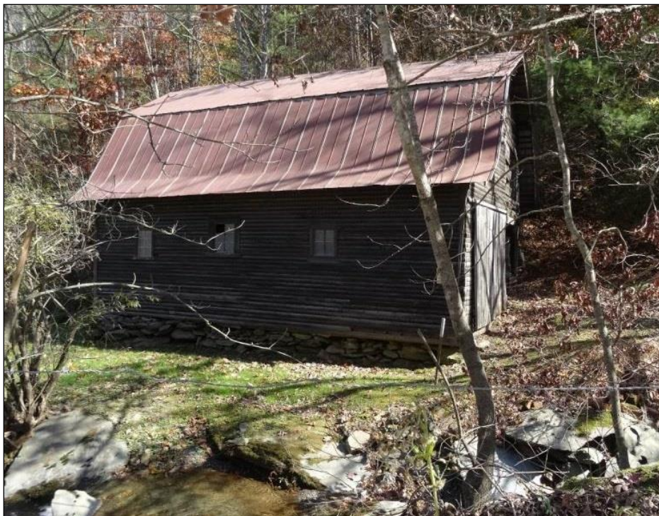
Photo 29: View of West Elevation of Barn across Clark's Creek.
