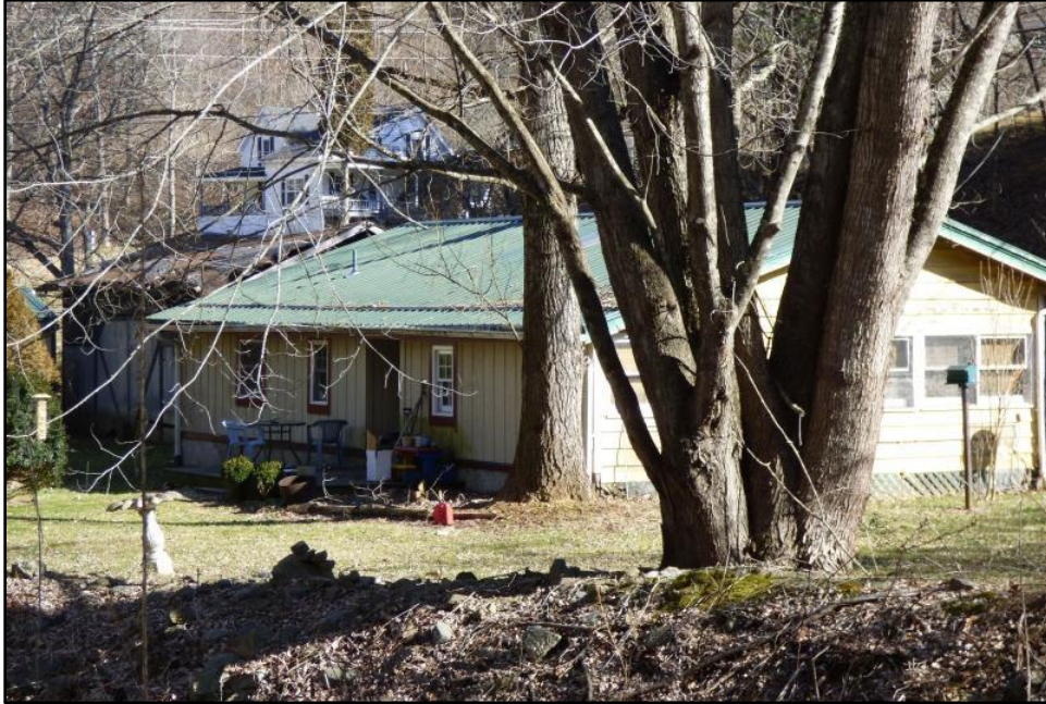
Photo 37: 157 Justus Road, West and South Elevations.
