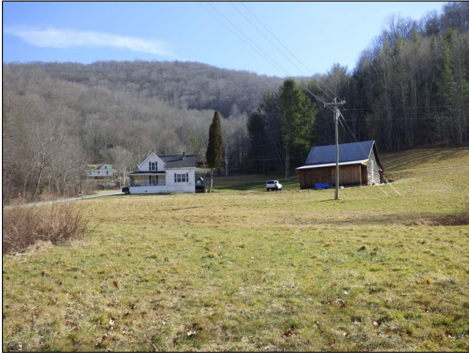
Photo 70: The Lowrance House and Barn, Looking West.
