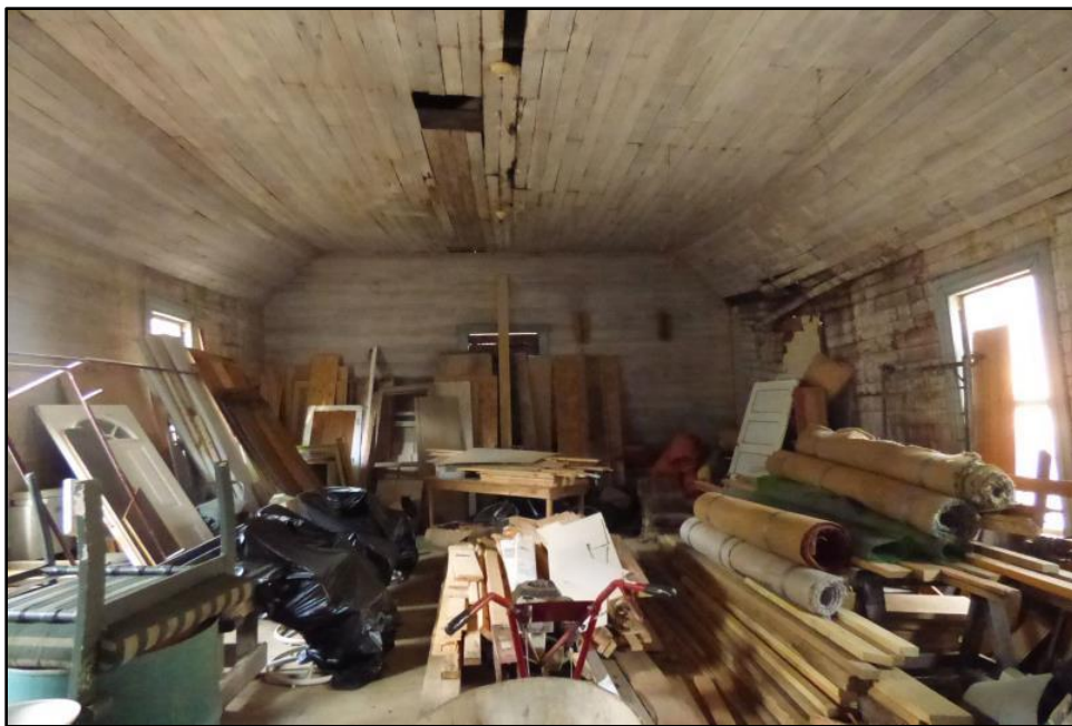
Photo 53: Clark's Creek Baptist Church, Interior, Looking North to Church Entrance Wall.
