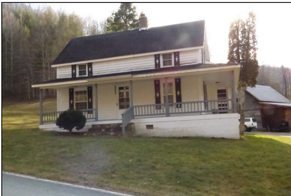
Photo 13: Lowrance House, Primary (North) Elevation, with Barn in Background.
