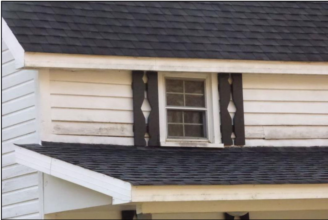
Photo 16: Lowrance House, Detail of Upper-Story Window (Replacement Sash).
