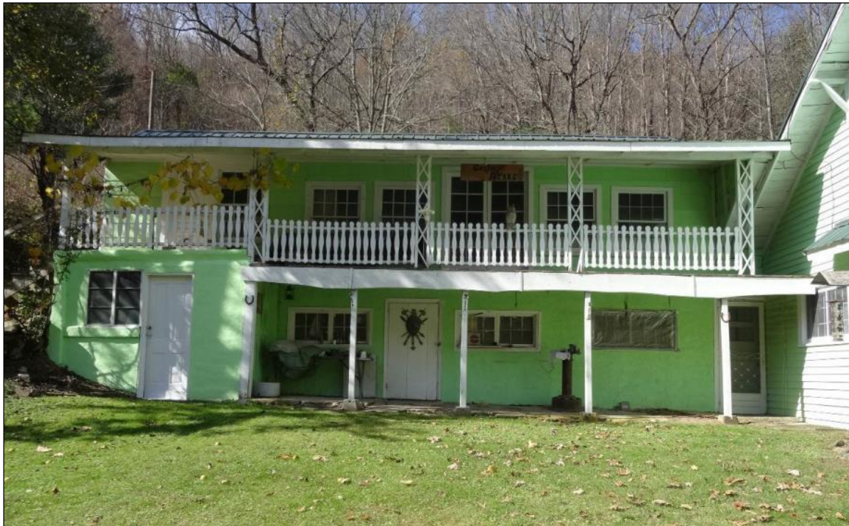
Photo 30: East Elevation of Cellar House and Loom Room (Second Floor).
