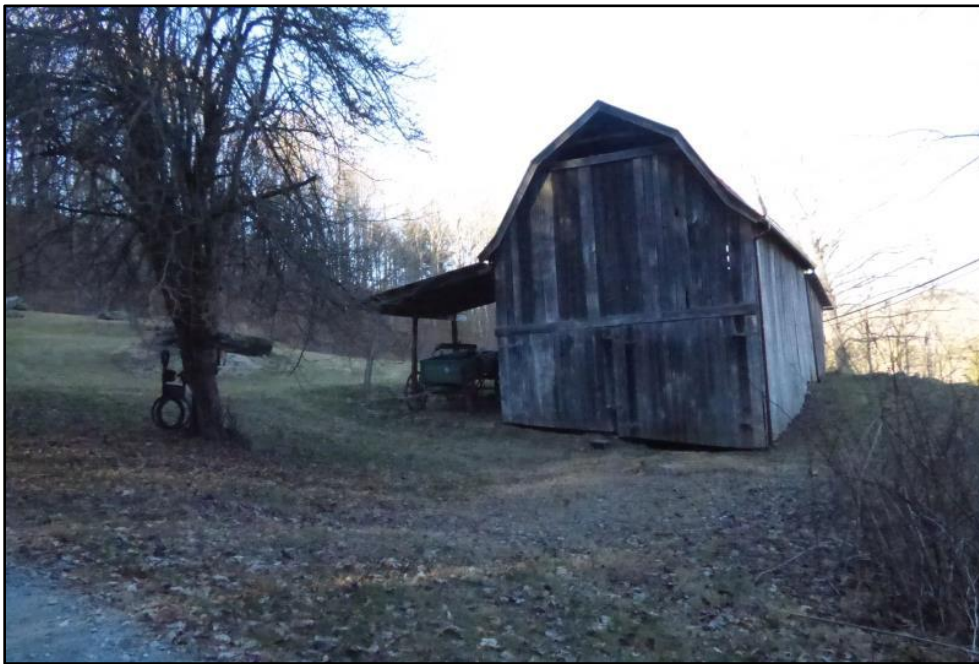
Photo 21: Barn, South Elevation with Pear Tree in Foreground.
