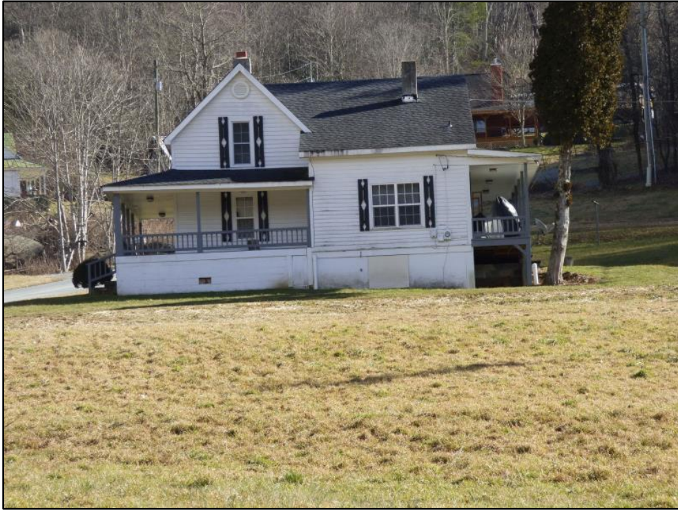
Photo 14: Lowrance House, West Elevation.
