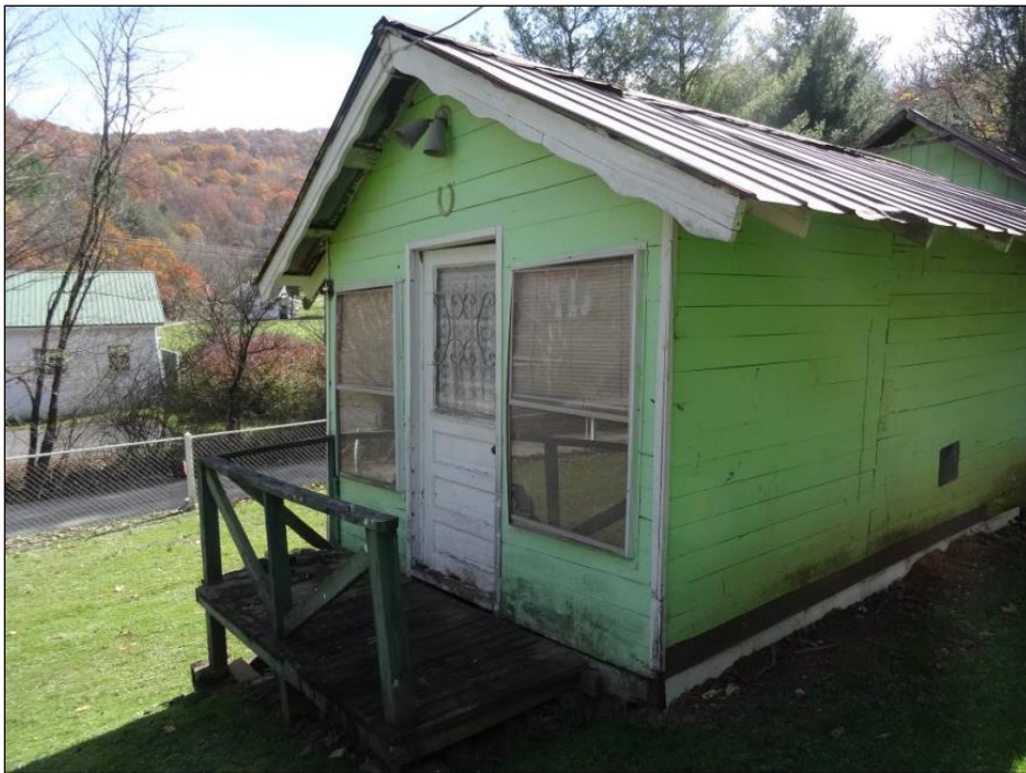
Photo 27: View of North Elevation of Workshop and Granary (Workshop).
