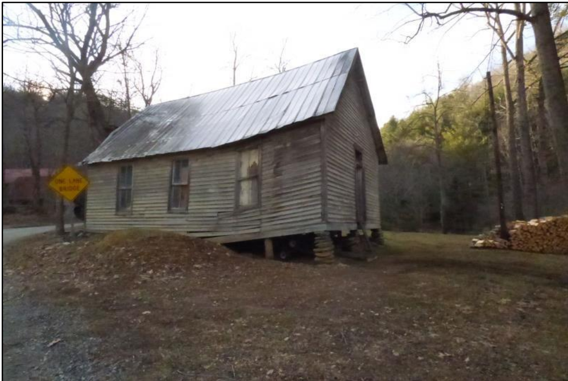
Photo 49: Clark's Creek Baptist Church, Oblique of East and Primary (North) Elevations.
