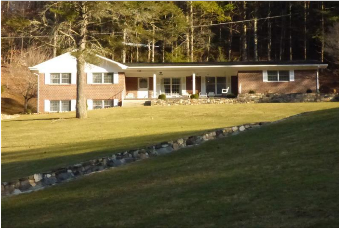
Photo 43: Johnny Byrd House, Primary (West) Elevation.
