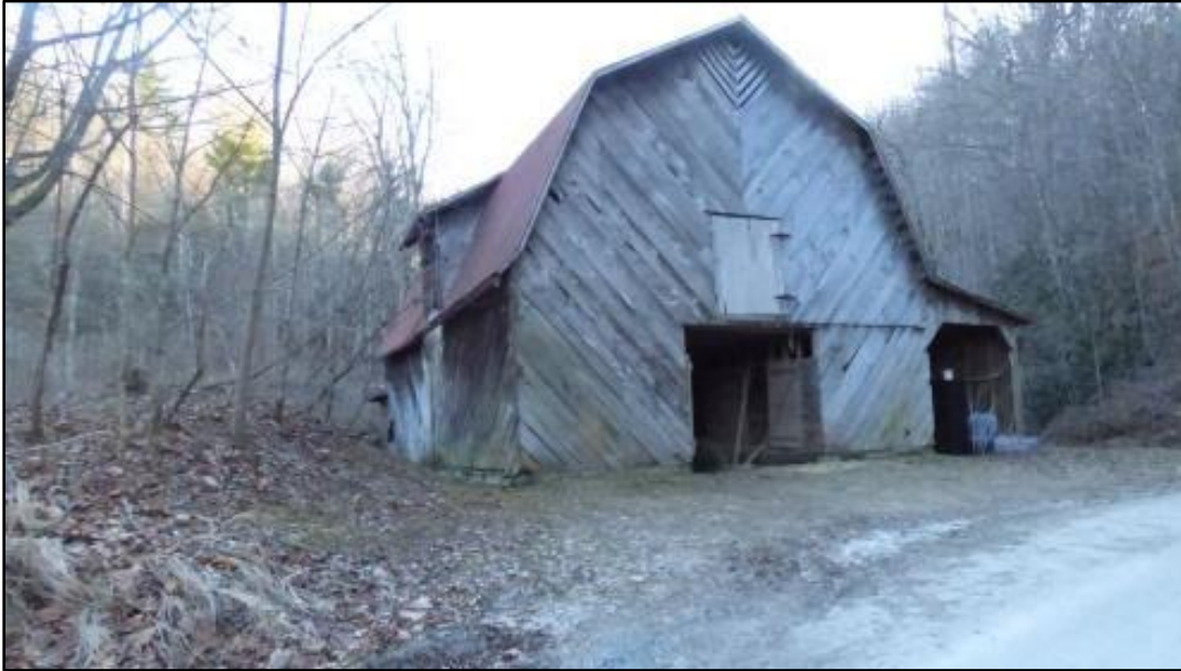
Photo 56: Barn, North Elevation.
