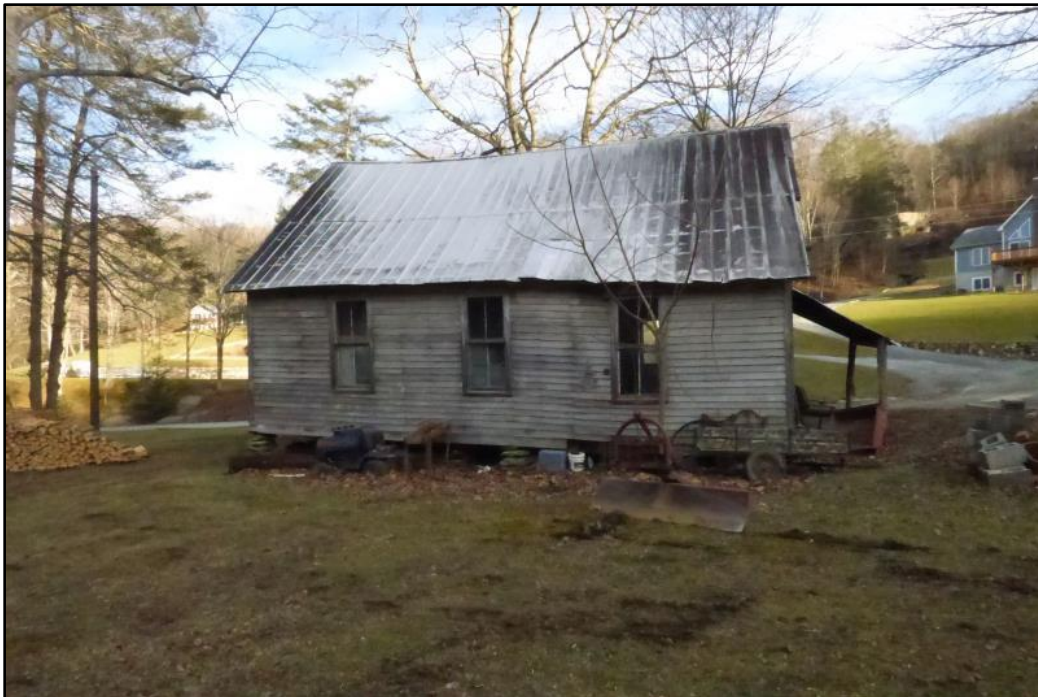
Photo 51: Clark's Creek Baptist Church, West Elevation.
