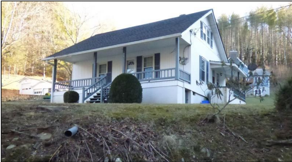
Photo 48: Wilson House, North and West Elevations.
