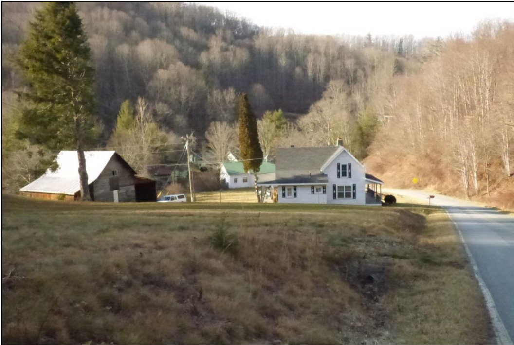
Photo 73: The Lowrance House and Barn, Looking East.
