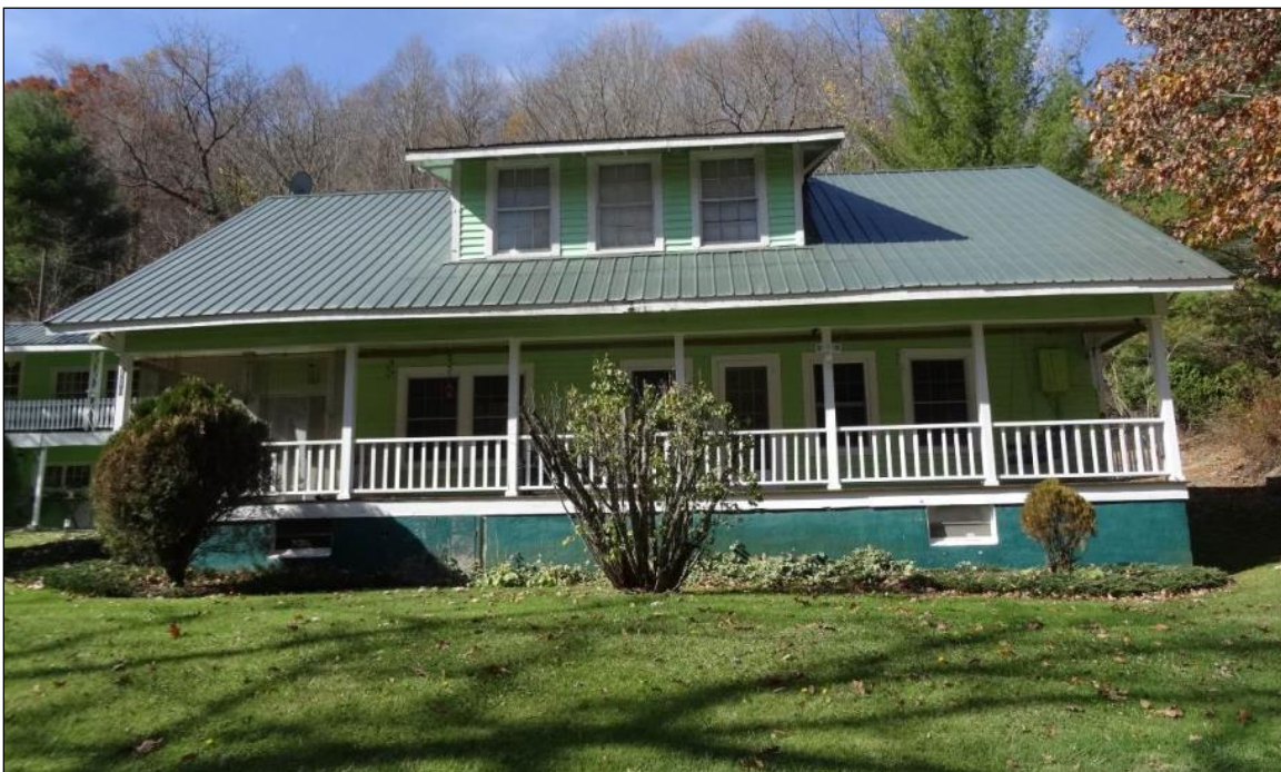
Photo 24: View of East Elevation and Porch Features, Clark House.
