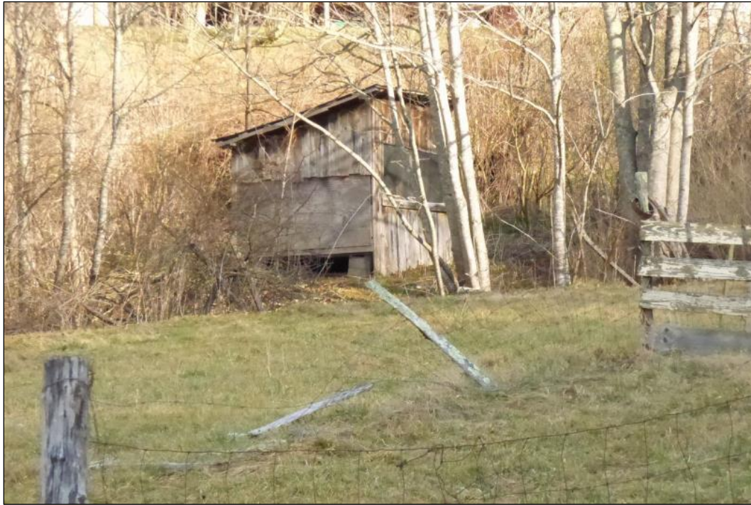
Photo 10: Moody Townsend House, South and East Elevations of Chicken Coop.
