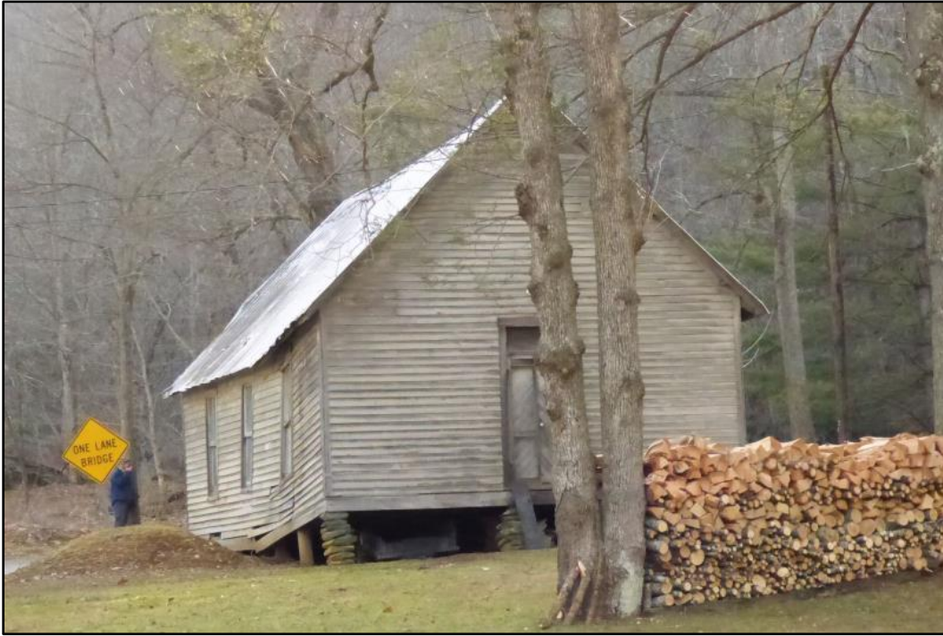
Photo 50: Clark's Creek Baptist Church, Partial Oblique of East and North Elevations.
