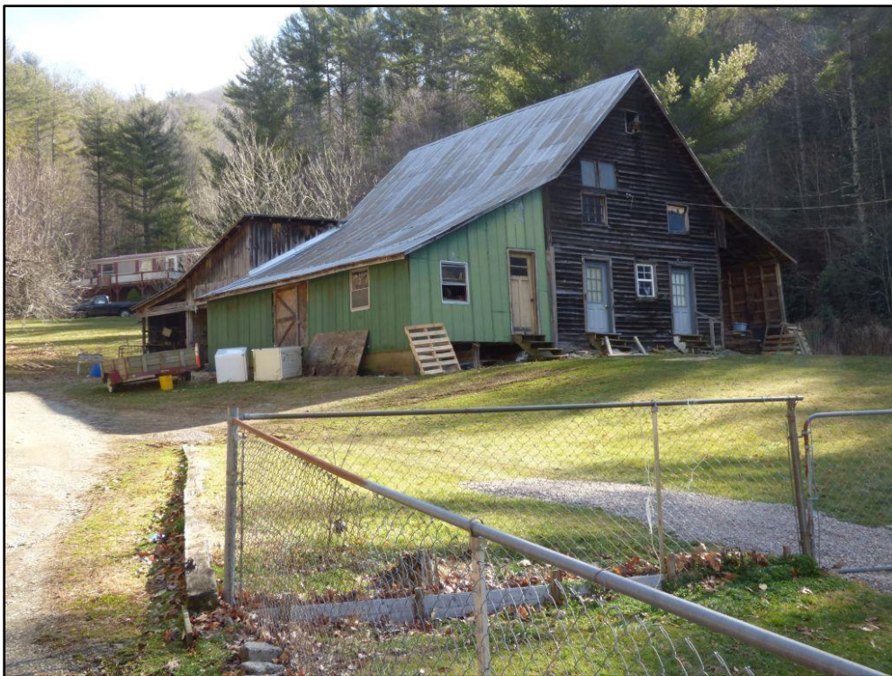
Photo 19: Pack House at 2840 Clark's Creek Road (Billy Townsend House, Not in Clark's Creek Rural Historic District). Oblique view of West and North (front) elevations.
