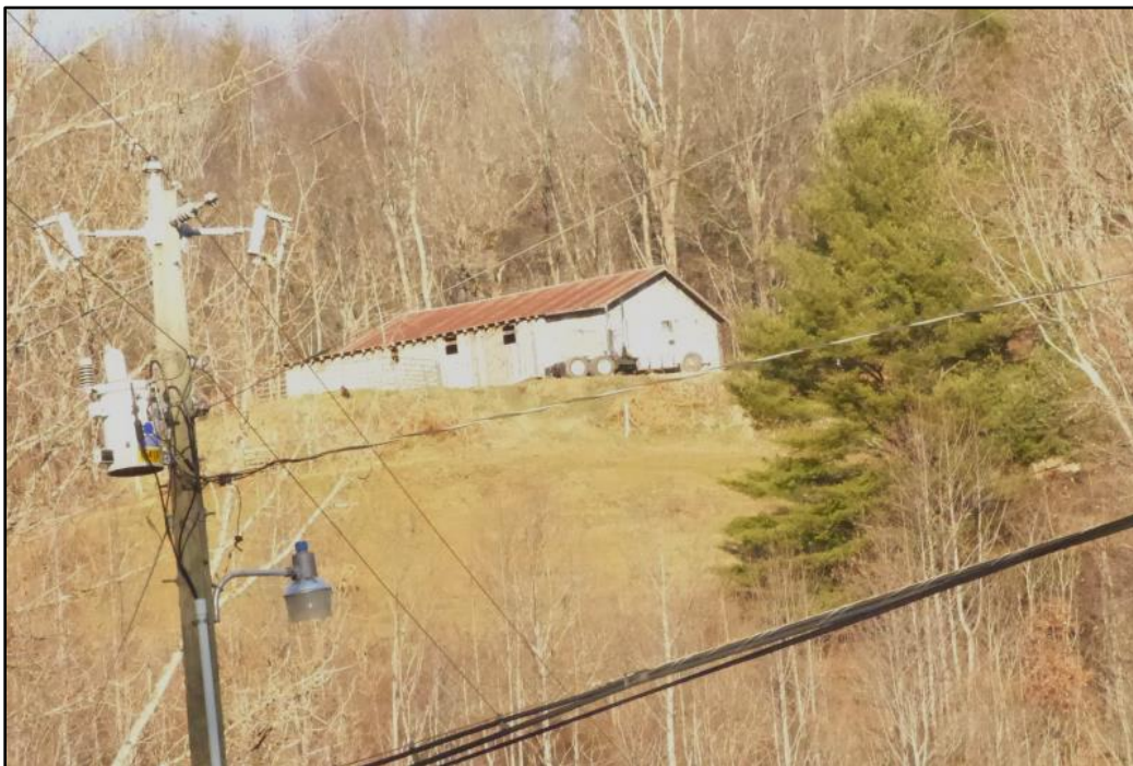
Photo 65: 2222 Clark's Creek Road, West and South Elevations of Barn.
