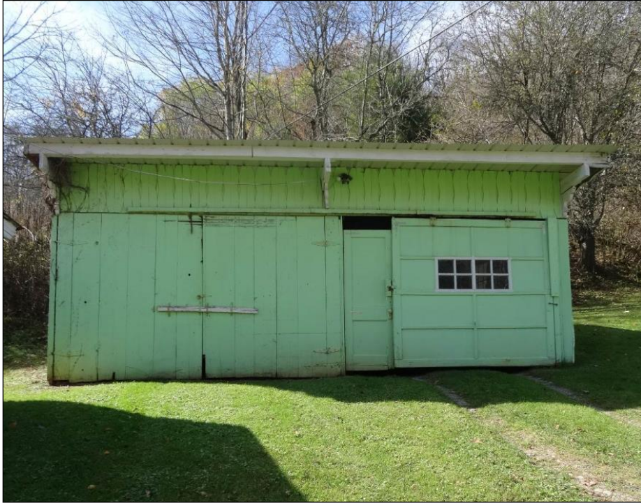
Photo 26: East Elevation of Garage.
