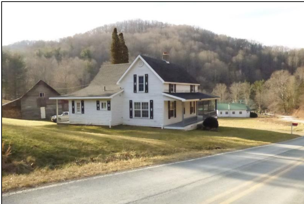
Photo 15: Lowrance House, Oblique of East and North Elevations.
